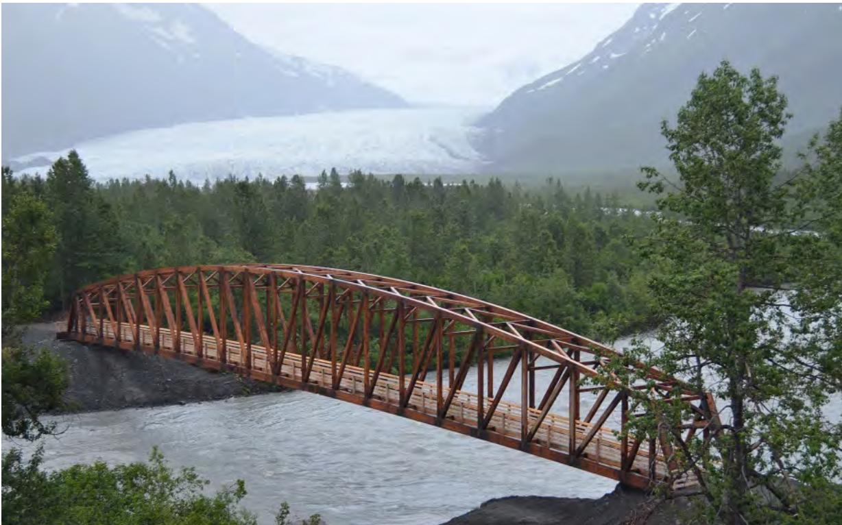
CAMELBACK TRUSS BRIDGE
