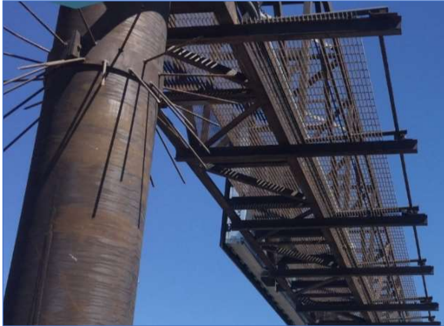
Photo 3. Example of galvanized steel treated with Natina Steel Solution.
