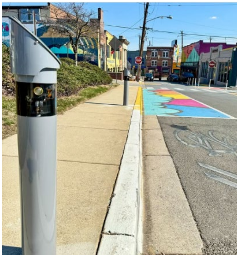
Figure 9: SafetySticks Installation in Hyattsville, Maryland
