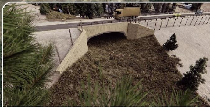
MP 193.0 - Arch Underpass
