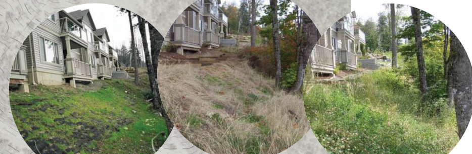
1 vegetated geomodular wall system
