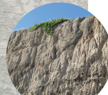
2 shotcrete retaining wall
