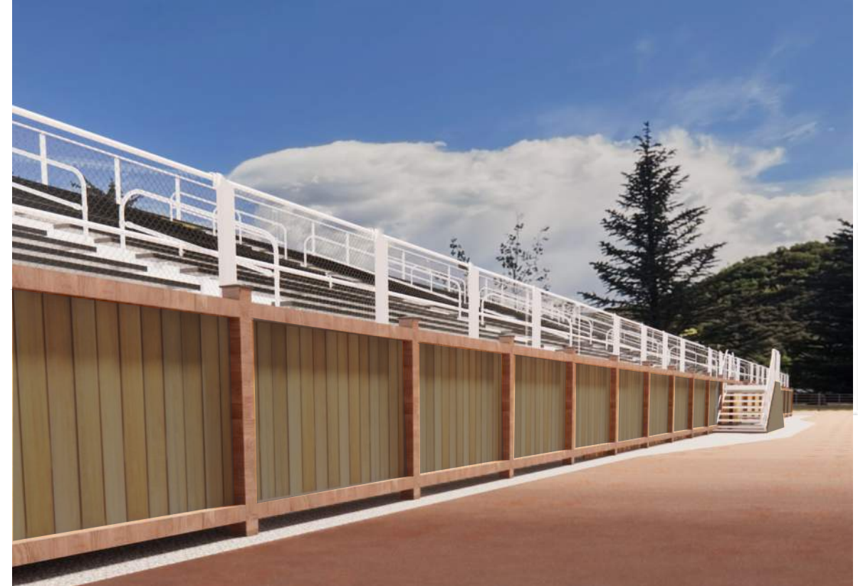
RE-FINISH FENCING PLANKS WITH GRAY-TONE SEMI-TRANSPARENT STAIN
