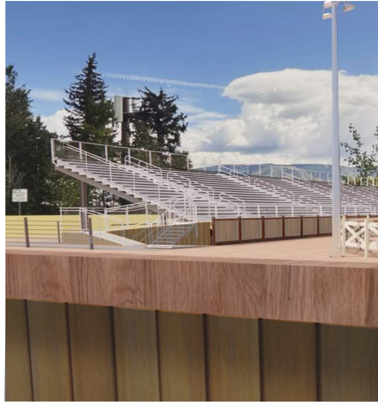
RE-FINISH FENCING PLANKS WITH GRAY-TONE SEMI-TRANSPARENT STAIN
