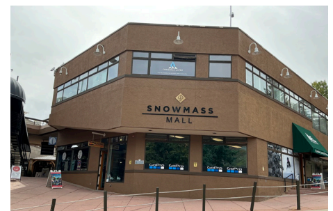
Figure 9. This is an example of a 'Building Identification Sign', as found in the definitions section of this document.
