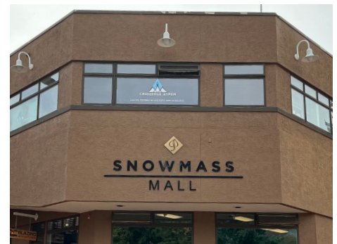
Figure 9. This is an example of a 'Building Identification Sign', as found in the definitions section of this document.
