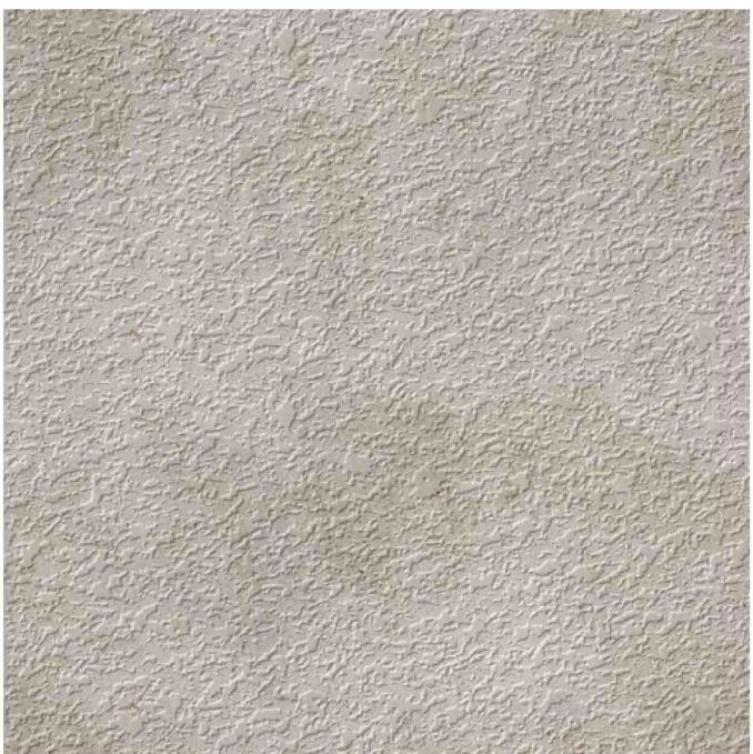
STUCCO SIDING B
