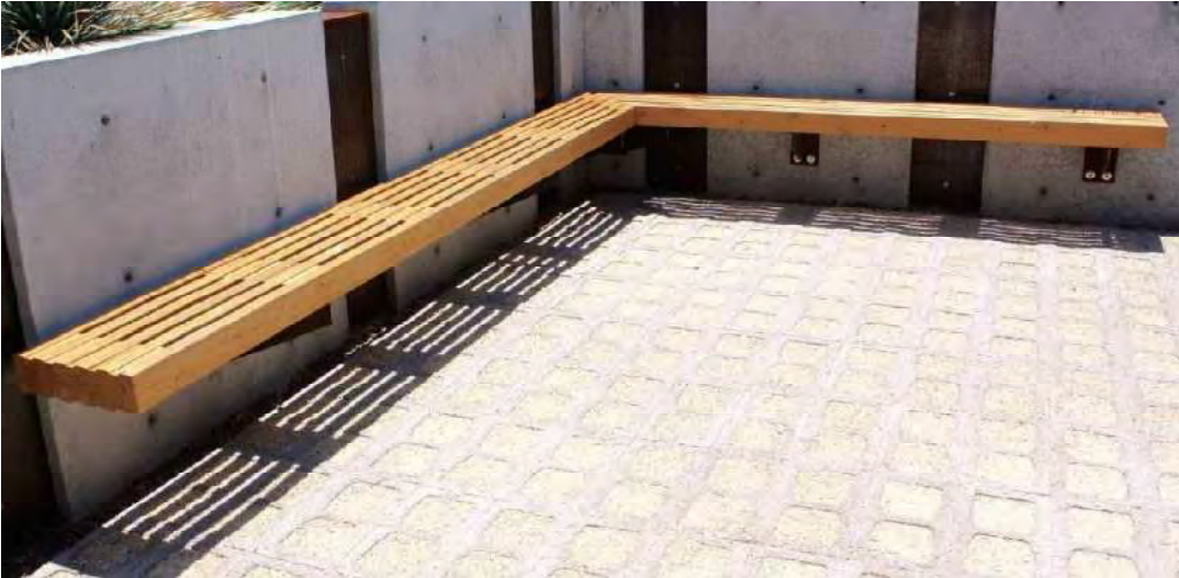
ATTACHED WOOD BENCH SEATING @ RAISED PLANTER
