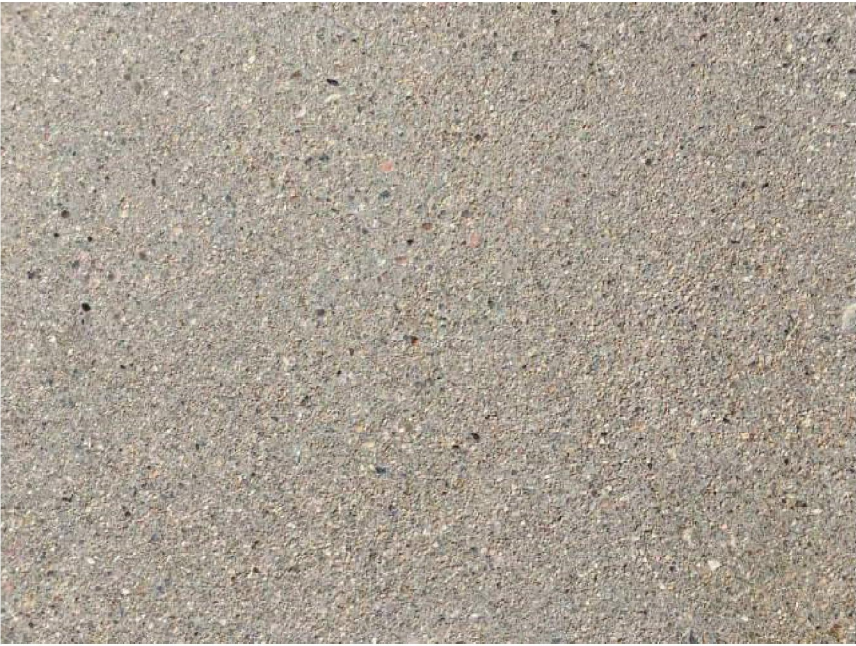
INTEGRAL COLOR CONCRETE PAVING WITH SAND FINISH
