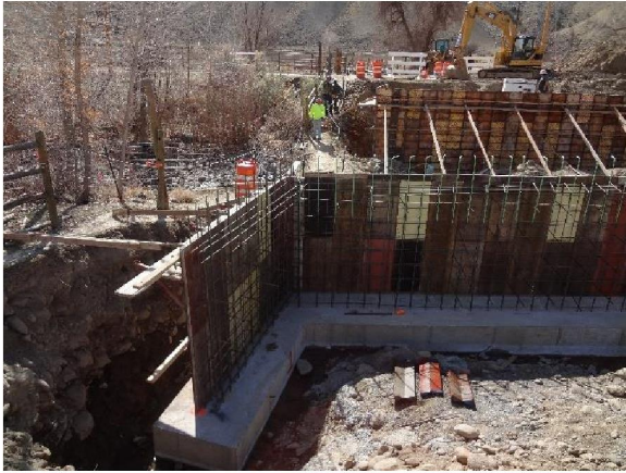
Abutments on Spread Footing
