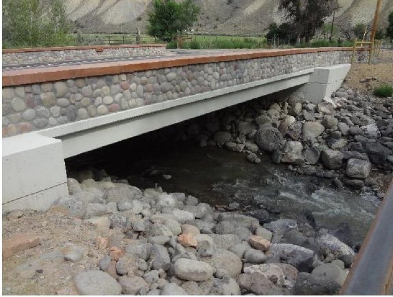
Bridge Example – Kannah Creek
