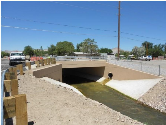
Bridge Example – D.5 Road over Lewis Wash
