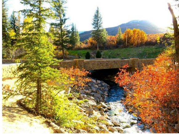
Bridge Example – 4 Mile Creek
