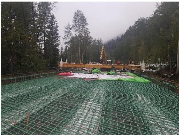
Reinforced Concrete Deck
