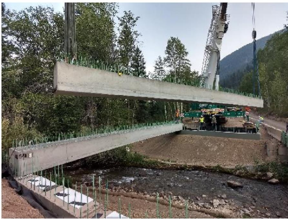
Precast/Prestressed Girders
