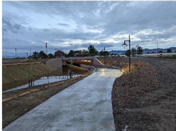
Bridge Example – G Road over N Leach Crk
