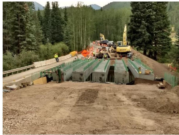
Precast/Prestressed Girders
