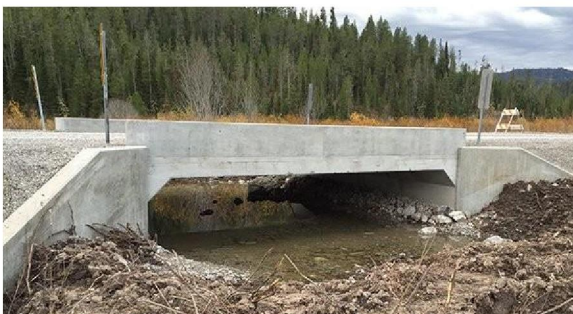
Oldcaslte 3-Sided Bridge - Idaho
