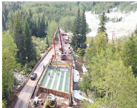
Deck Placement/Finishing
