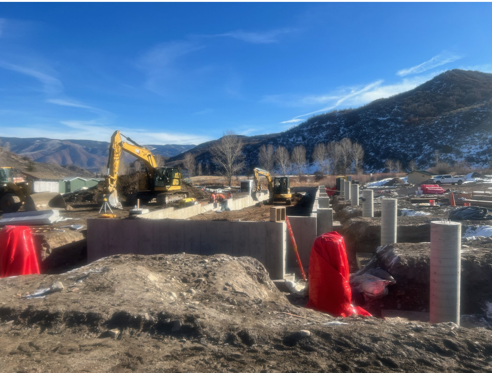
November 30 Concrete poured and curing
