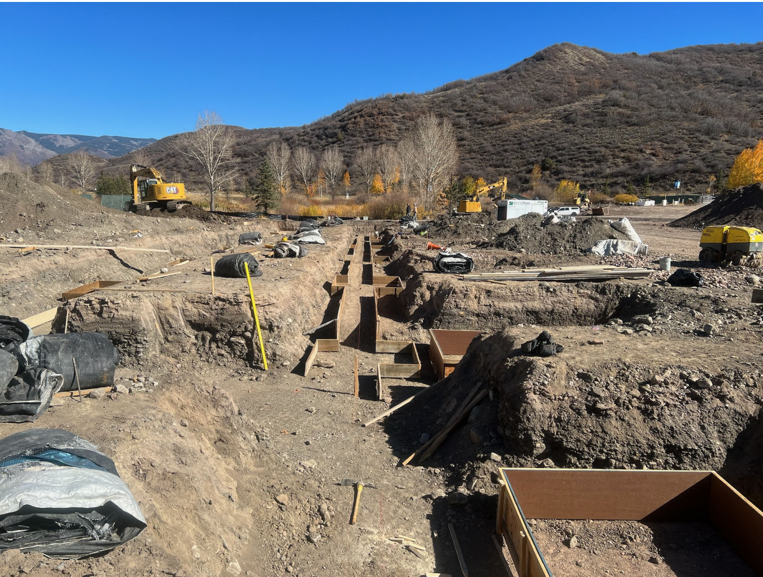
October 25 Framing before concrete
