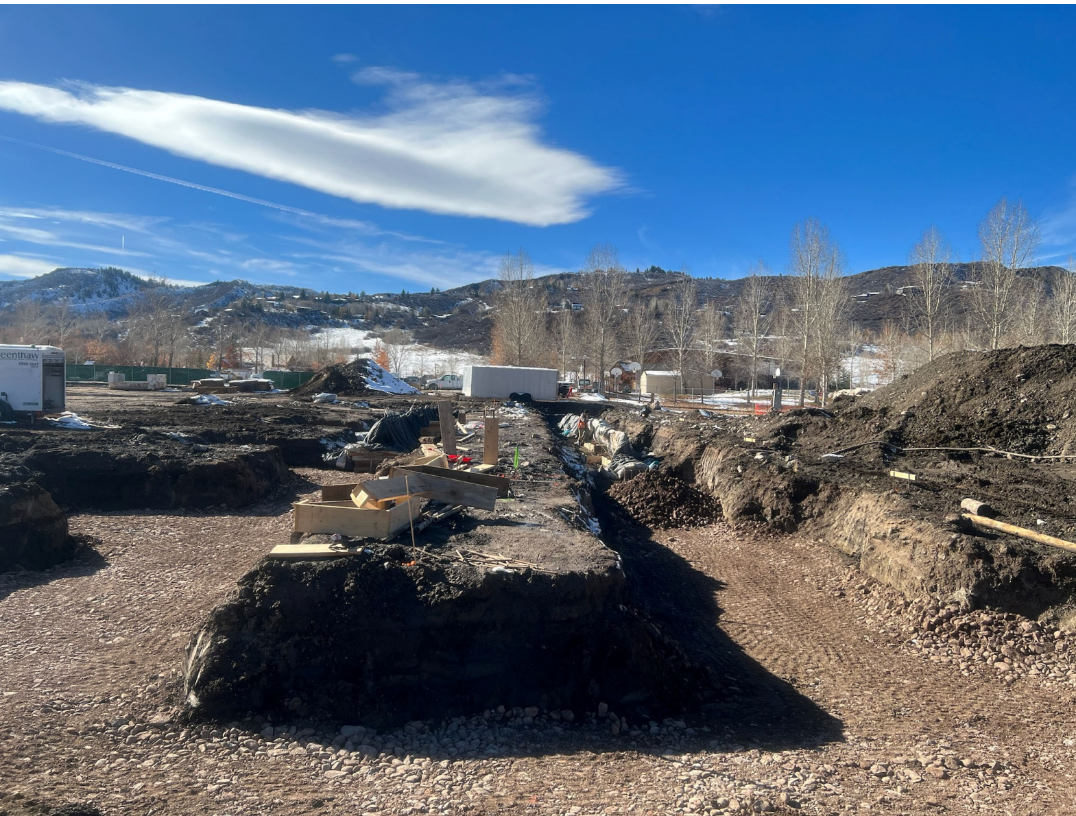
November 1 Foundation being laid
