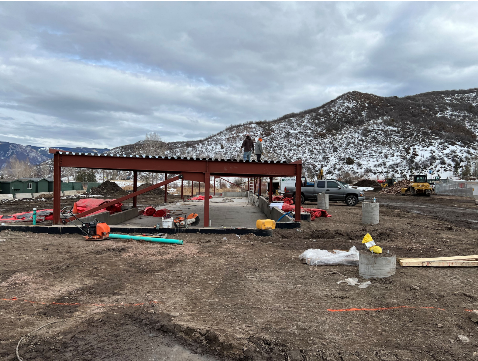
December 19 Structure frame installed
