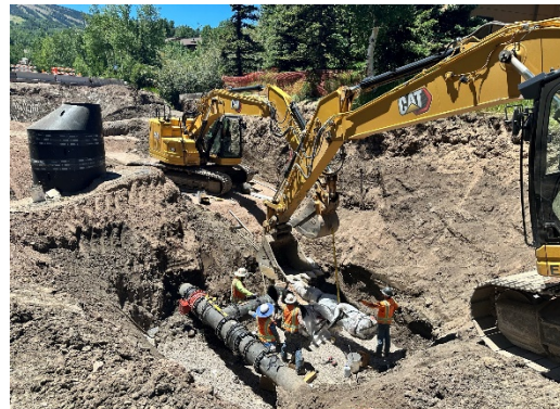
Water line tie-in
