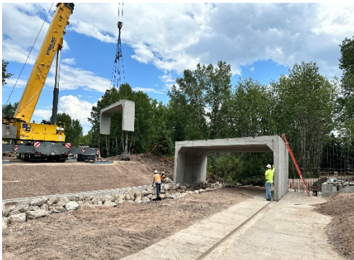
Precast structure placement
