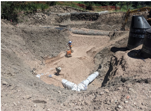
Relocated Water line being backfilled
