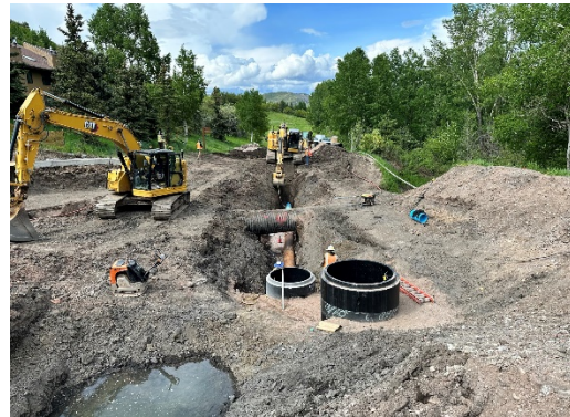
Relocated Sewer line under temp creek pipe
