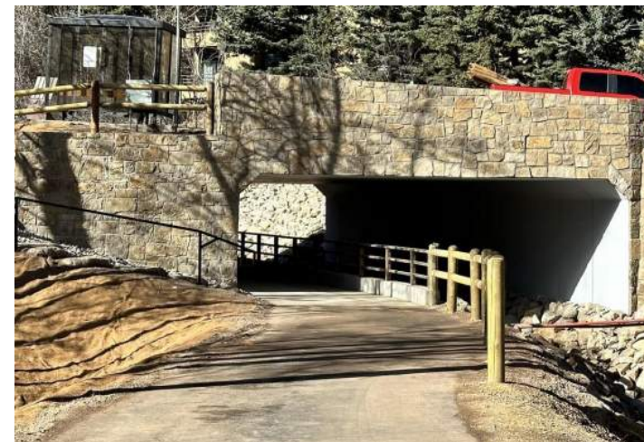
WALL (CAST IN PLACE CONCRETE WITH STONE VENEER FROM BRUSH CREEK CULVERT)
