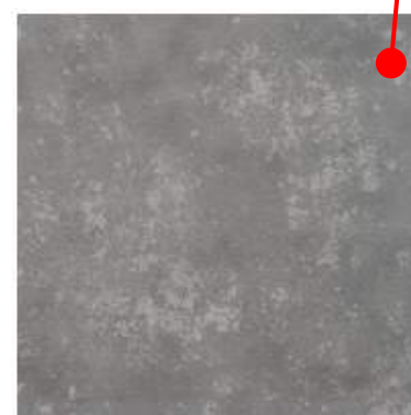
EXPOSED CONCRETE AT SITE AND SUBGRADE GARAGE FOUNDATION WALLS
