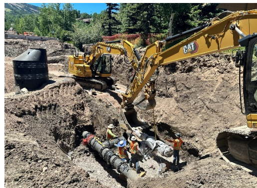
Water line tie-in
