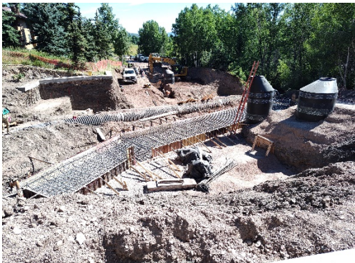
South abutment footing ready for concrete
