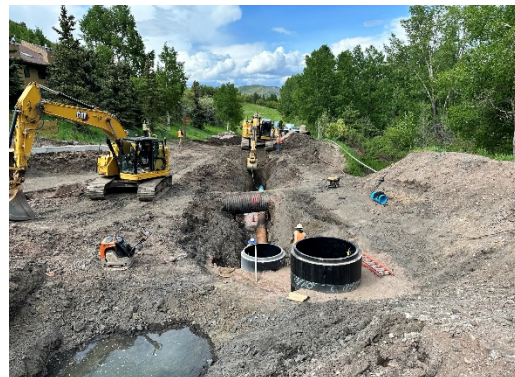
Relocated Sewer line under temp creek pipe
