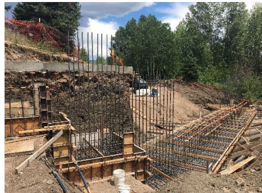
North abutment footing ready for concrete
