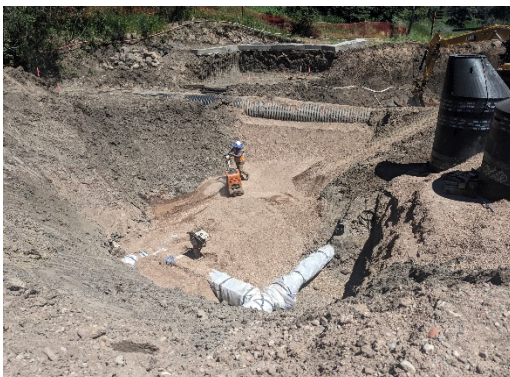
Relocated Water line being backfilled
