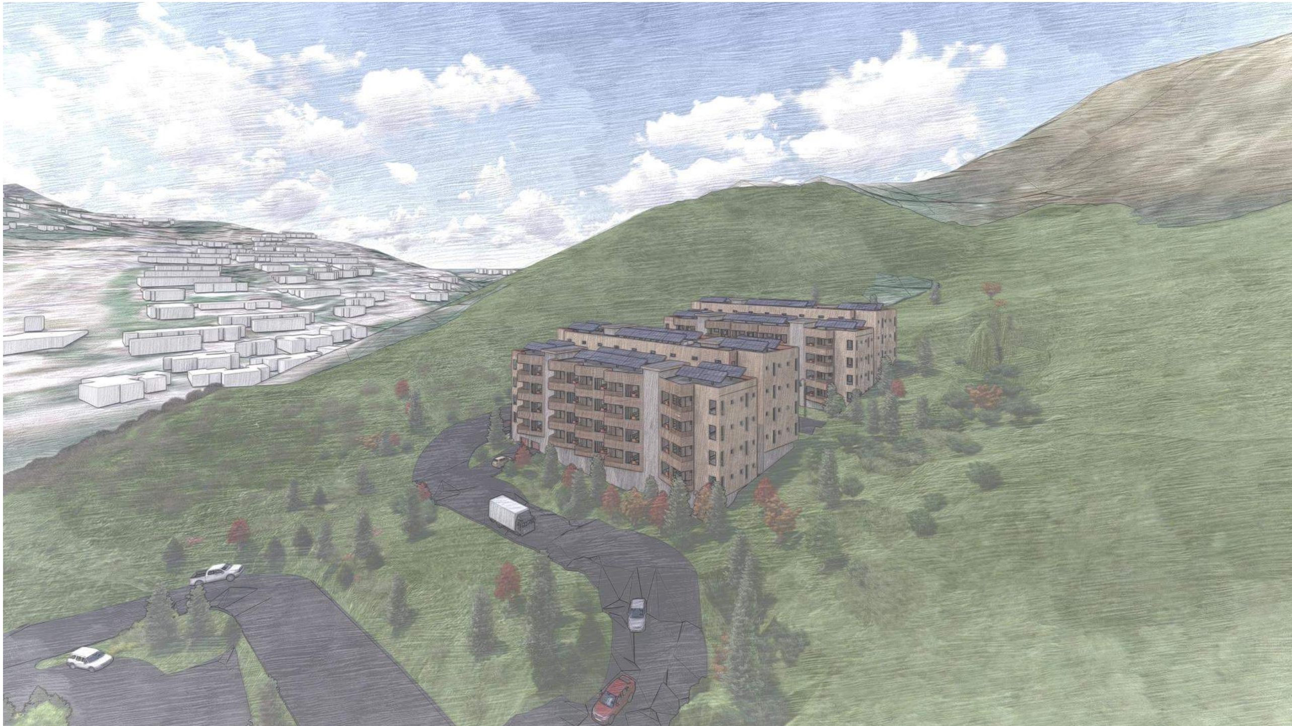
aerial site view
