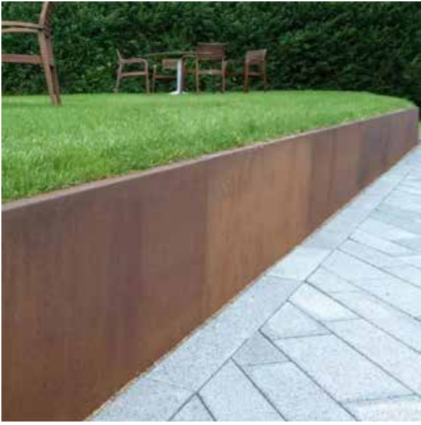
Blending grading and creating flat spaces for recreation using steel retaining walls
