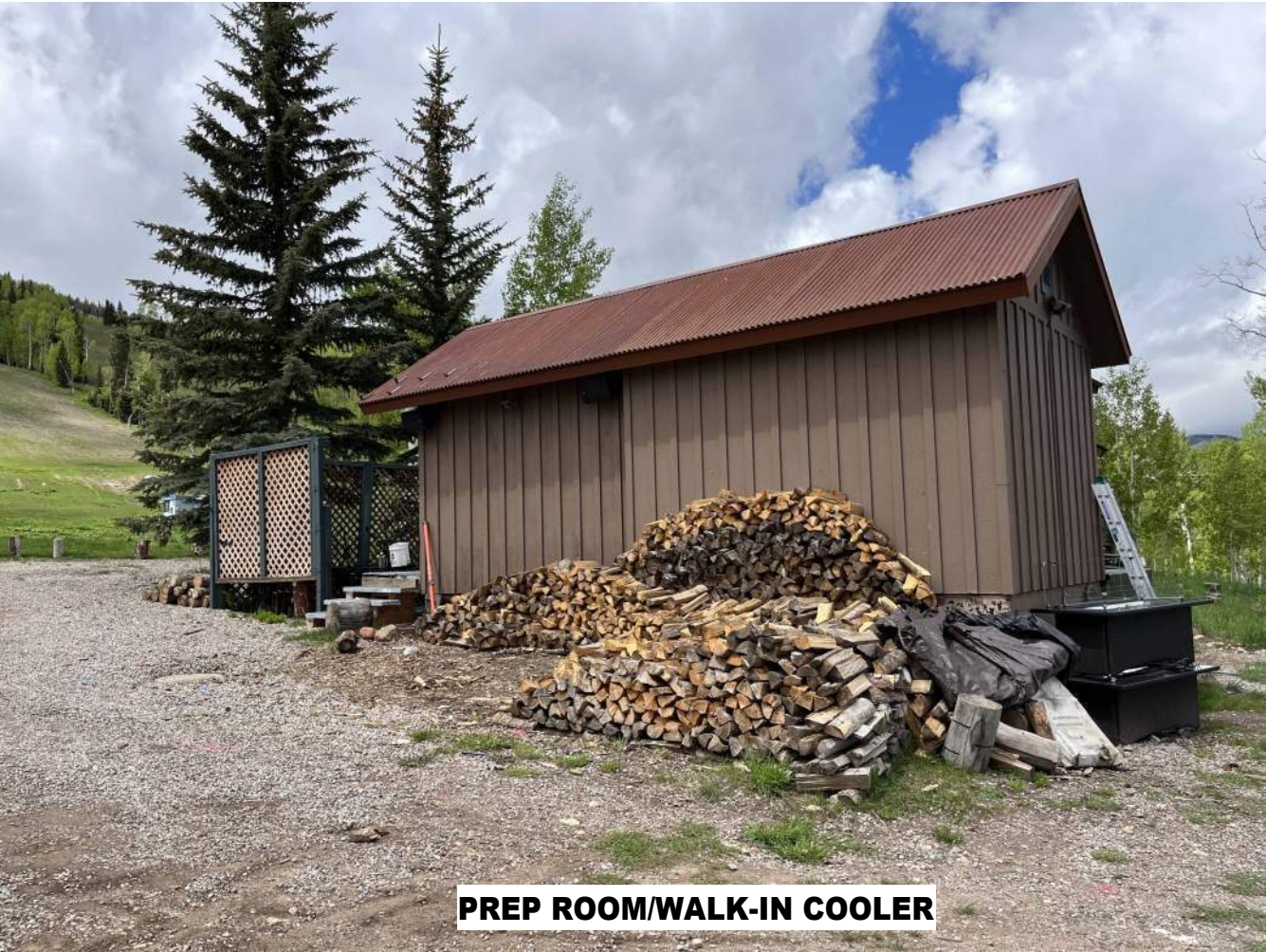
PREP ROOM/WALK-IN COOLER
