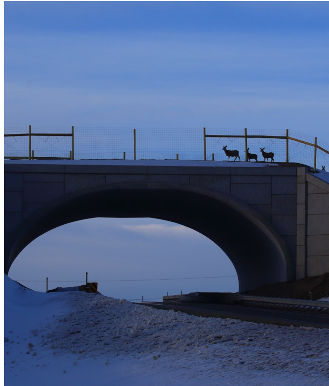
SH 9, Grand County Colorado
