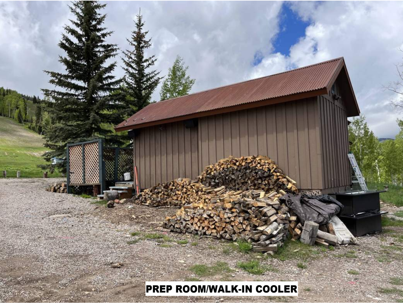
PREP ROOM/WALK-IN COOLER
